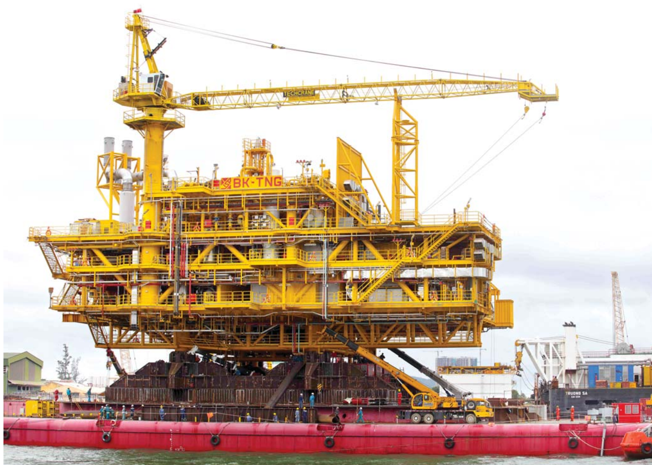
Load-out of BK-Thien Ung platform topside. Photo: Duc Hau
